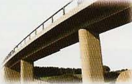
a concrete bridge
